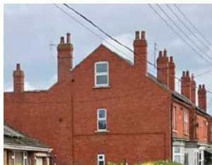
Figure 107: Edwardian chimney stacks.
