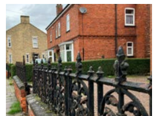
Figure 70: Brick wall and metal railings.
