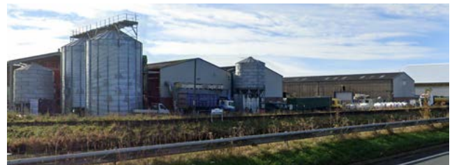
Figure 189: Industrial Saxilby opposite the Fossdyke Canal as viewed from Lincoln Road.
