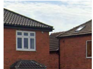
Figure 99: Industrial red brick.
