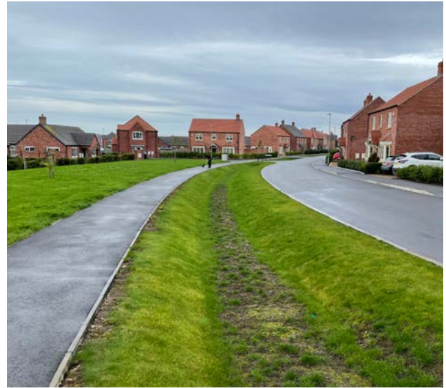
Figure 166: Sustainable drainage systems (SuDS) include swales.
