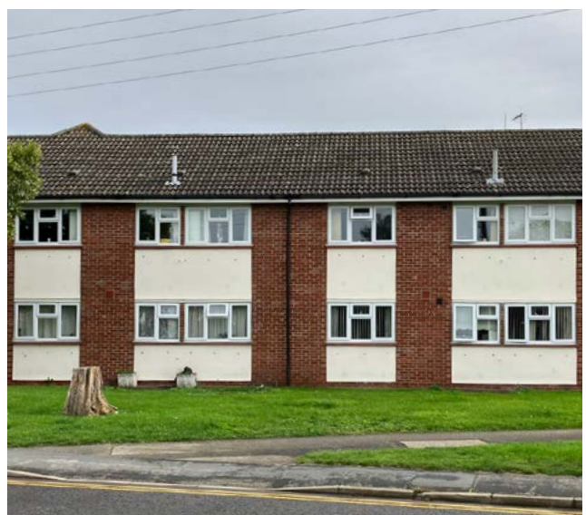
Figure 42: The large blocks containing flats between High Street and Manor Road.
