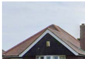
Figure 86: Pitched roofs and chimney stacks.
