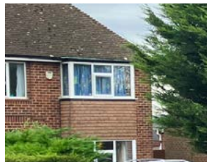
Figure 87: Suburban bay windows.
