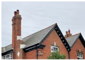
Figure 65: Pitched roofs and chimney stacks.
