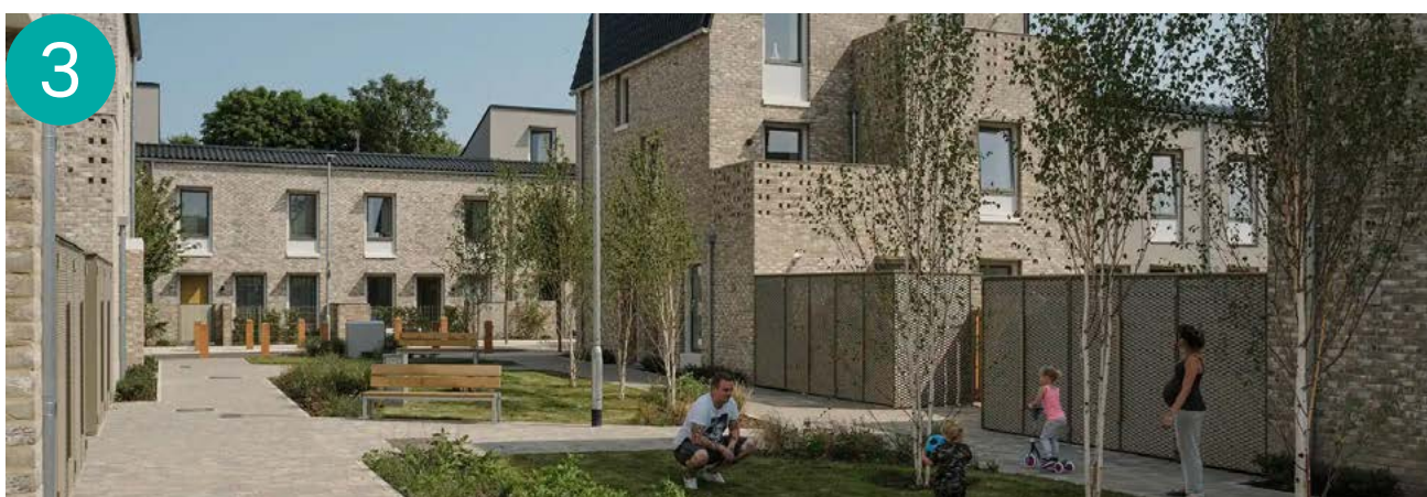
Figure 206: Innovate: This development on Goldsmith Street in Norwich won the 2019 Stirling Prize. The development creates a gentle level of density in a modern interpretation of terraced housing. Sustainability is a priority with roofscapes modelled to the winter sun angle and with full solar design. Streets are pedestrian friendly and there is an emphasis on tree planting and public spaces. Despite the innovative design, the use of brick and vertical windows is still recognisably part of the local vernacular and the development blends in well to its surroundings.
