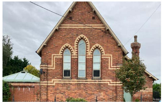
Figure 44: The former Mission Church of St Andrew, now a private home.
