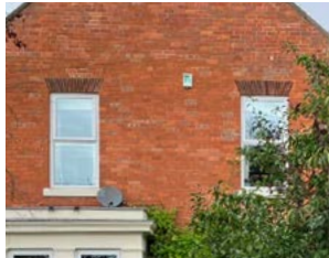
Figure 64: Industrial red brick.
