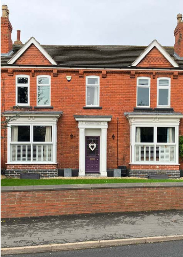
Figure 14: Saxilby's Edwardian heyday is evident in its architecture.
