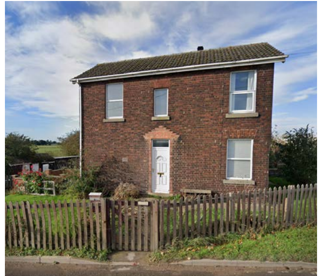
Figure 193: The railway crossing house on Saxilby Road.
