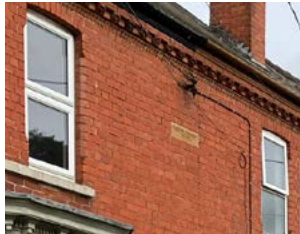
Figure 106: Industrial red brick.
