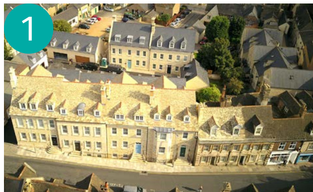
Figure 204: Harmonise: New development (centre, left and back) in Stamford, Lincolnshire which successfully imitates the historic buildings to the right and opposite. The buildings are neo-Georgian using local building and roofing materials. The modest setback gives an indication that these are recent additions, but otherwise the historic streetscape has been restored.
