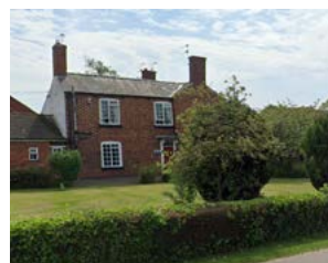
Figure 90: Large front gardens.
