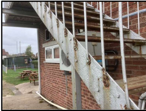
Figure 1: Right Hand Fire Escape
