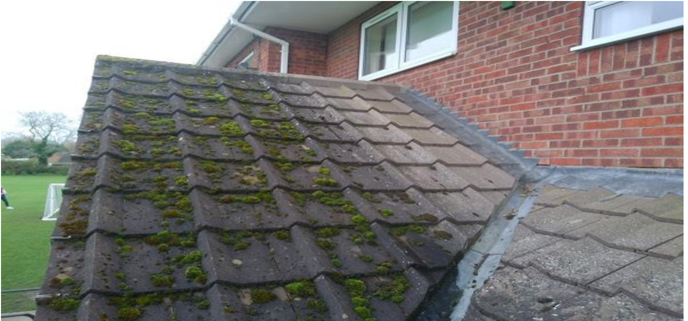
Porch roof area
