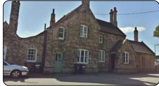
Railway Station and House (Grade II)
