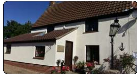
Saxilby Old Hall (Grade II*)
