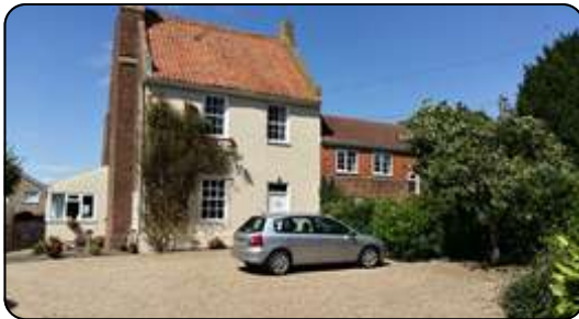
The Manor Farmhouse (Grade II)
