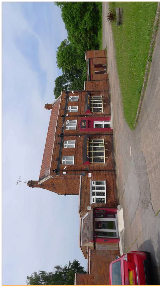
Figure 5.17: The inter-war former Bridge Inn building.
