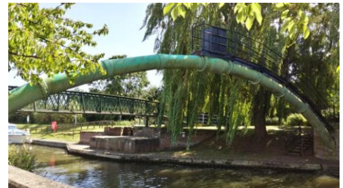
Pipe Bridge, Canal Footbridge and Abutment
