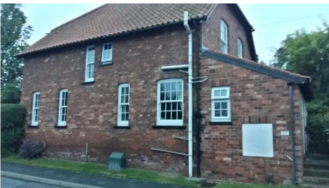
Former Farmhouse, 37 Church Road
