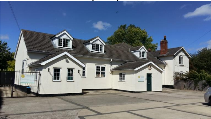
Former National C of E School, Church Lane (1845)
