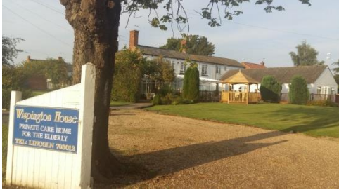
Wispington House, Mill Lane
